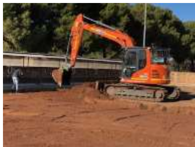
Removing the original soil
