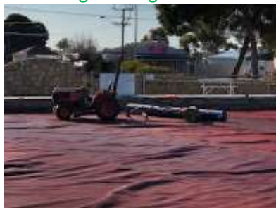
Laying the base cover
