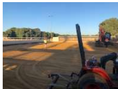
levelling the dumped sand/soil
