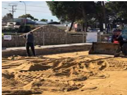
Starting to level the sand/soil
