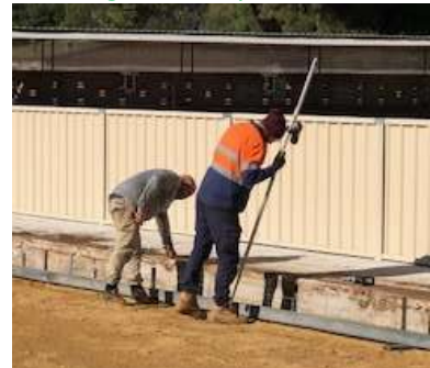
Preparing the plinth for the edges
